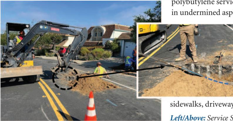
The Hastings Drive Service Connection Replacements Project improves system reliability and updates the existing service connection materials to current standards. Finishing of the project included restoration of sidewalks, driveways, slurry seal of streets, and striping. ■
