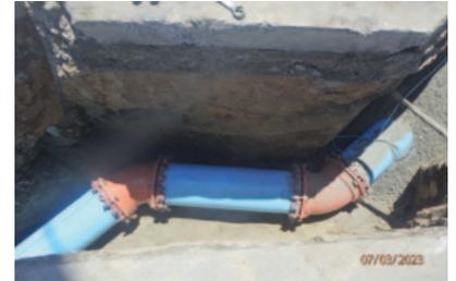
The District has experienced several leaks on the existing Harbor Boulevard water main, installed in 1967. Harbor is a highly traveled roadway serving local businesses in addition to on/off ramps to Highway 101 and leaks along this particular stretch of roadway are not ideal. This project replaces the existing water main with a new 12" polyvinyl chloride (PVC).
