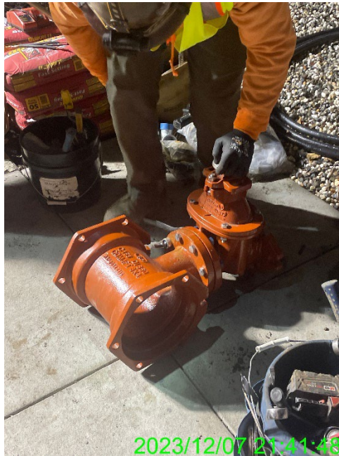
Valve Installation, December 7, 2023 , Old County Road
