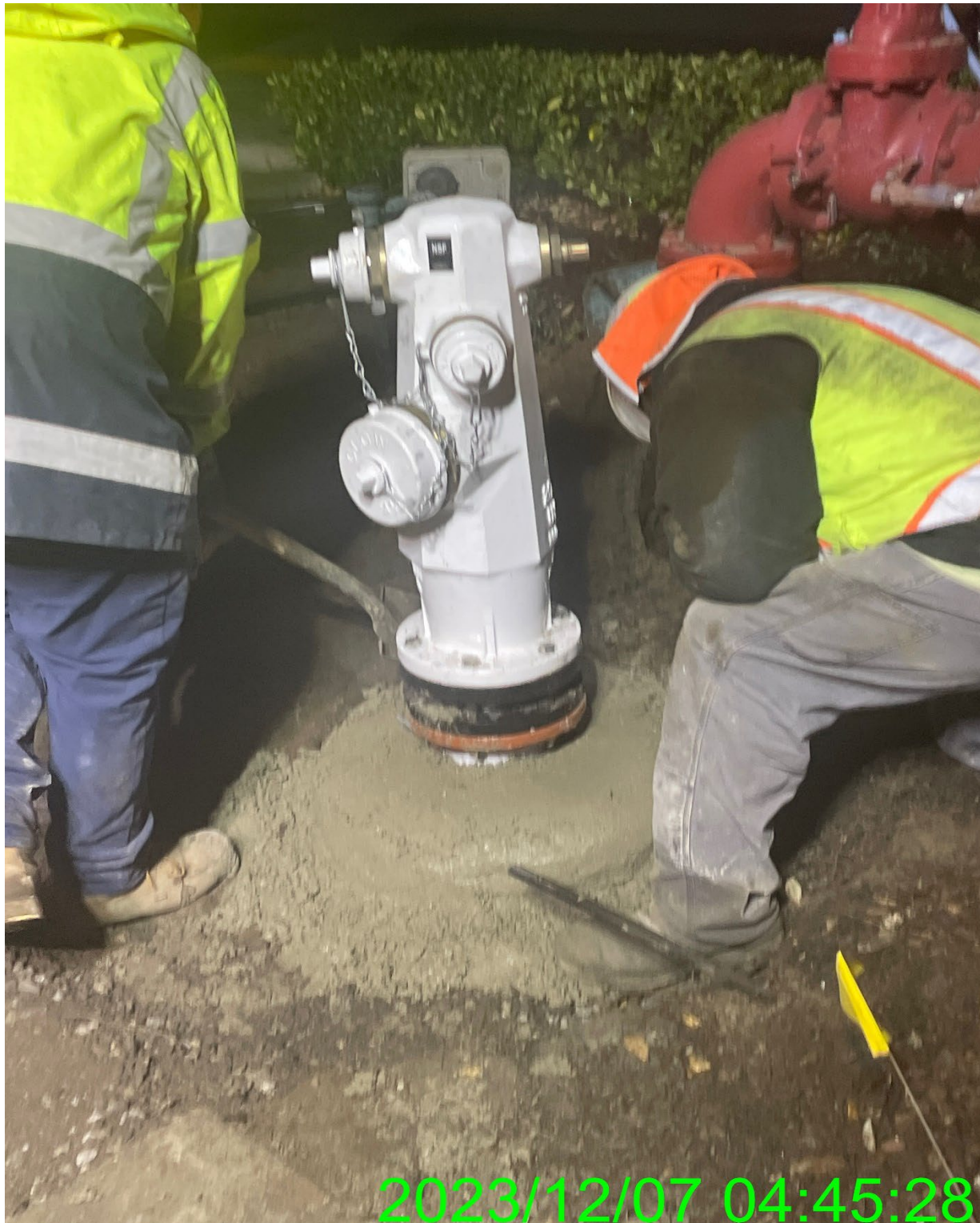
New hydrant install, December 7, 2023, Old County Road
