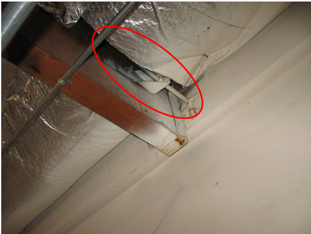
Photo 24: Typical Roof to Wall Tie
