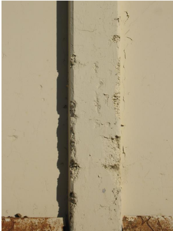
Photo 6 and 7: Rock Pockets and Damage at Concrete Pilasters
