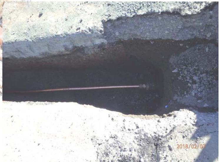
February 7, 2018—Service lines (Mezes Ave)
