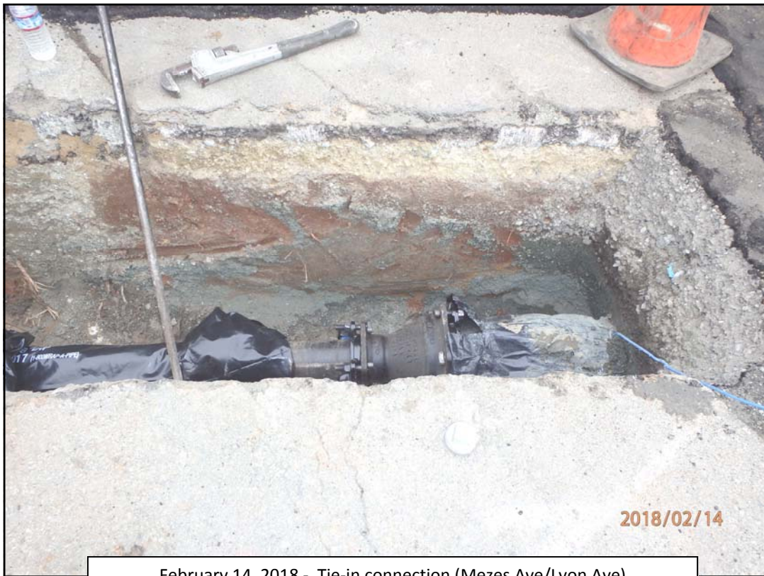
February 14, 2018 - Tie-in connection (Mezes Ave/Lyon Ave)
