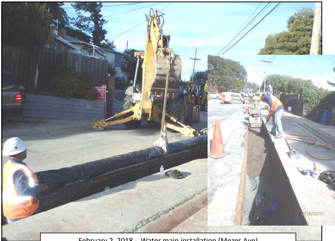
February 2, 2018 - Water main installation (Mezes Ave)
