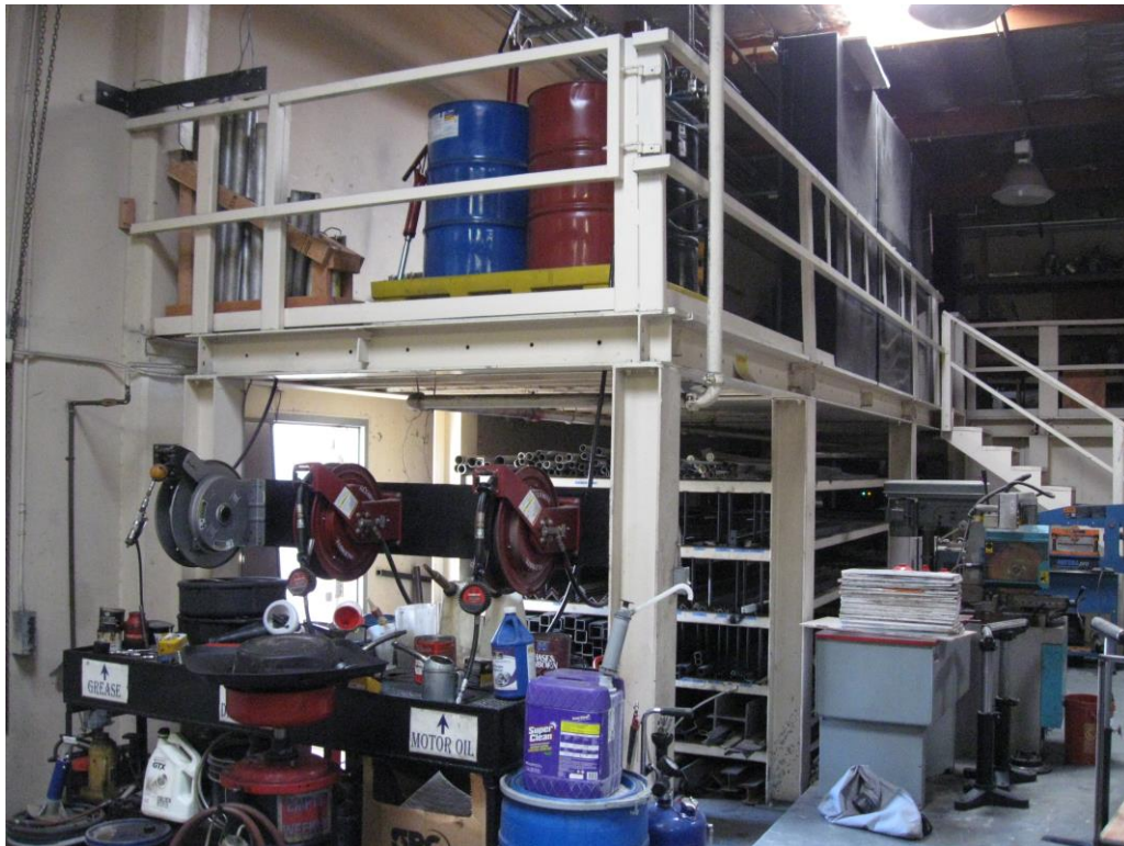
Photo 17b: Steel Framed Mezzanine
