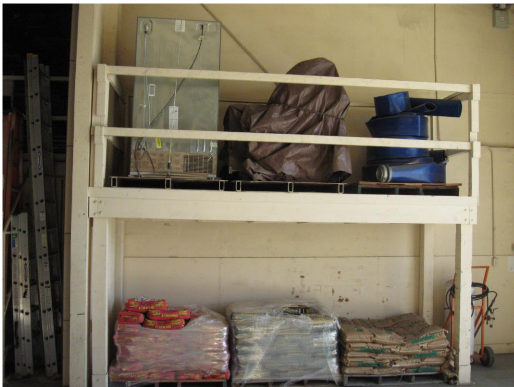
Photo 17a: Typical Wood Frame Mezzanine
