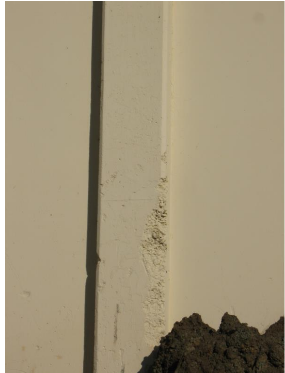
Photo 6 and 7: Rock Pockets and Damage at Concrete Pilasters
