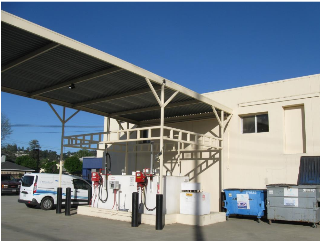
Photo 20: Exterior Steel Canopy
