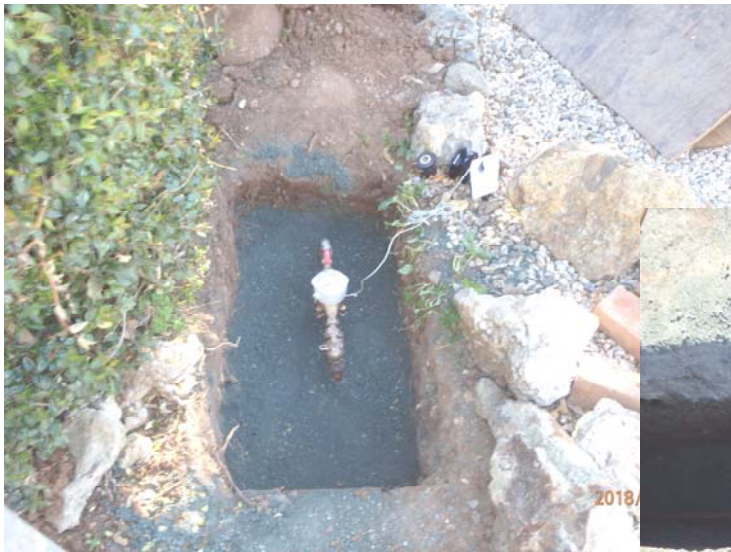
February 7, 2018—Hand digging for service connections (Mezes Ave)
