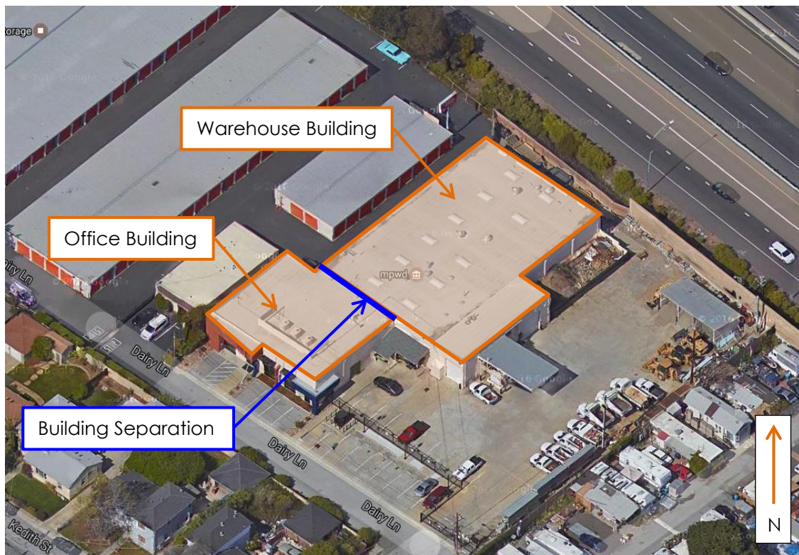
Figure 1: Aerial View of Headquarters Building
