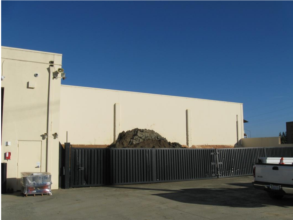
Photo 5: Side Storage Yard
