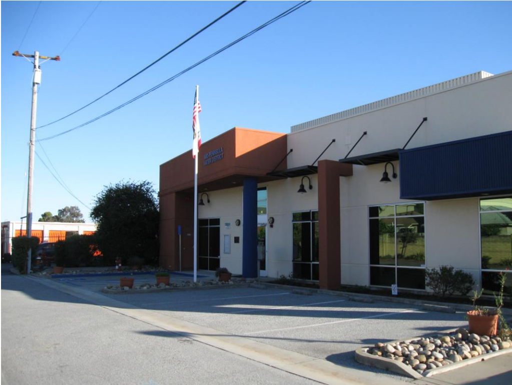
Photo 1: Front Entry of Office Building
