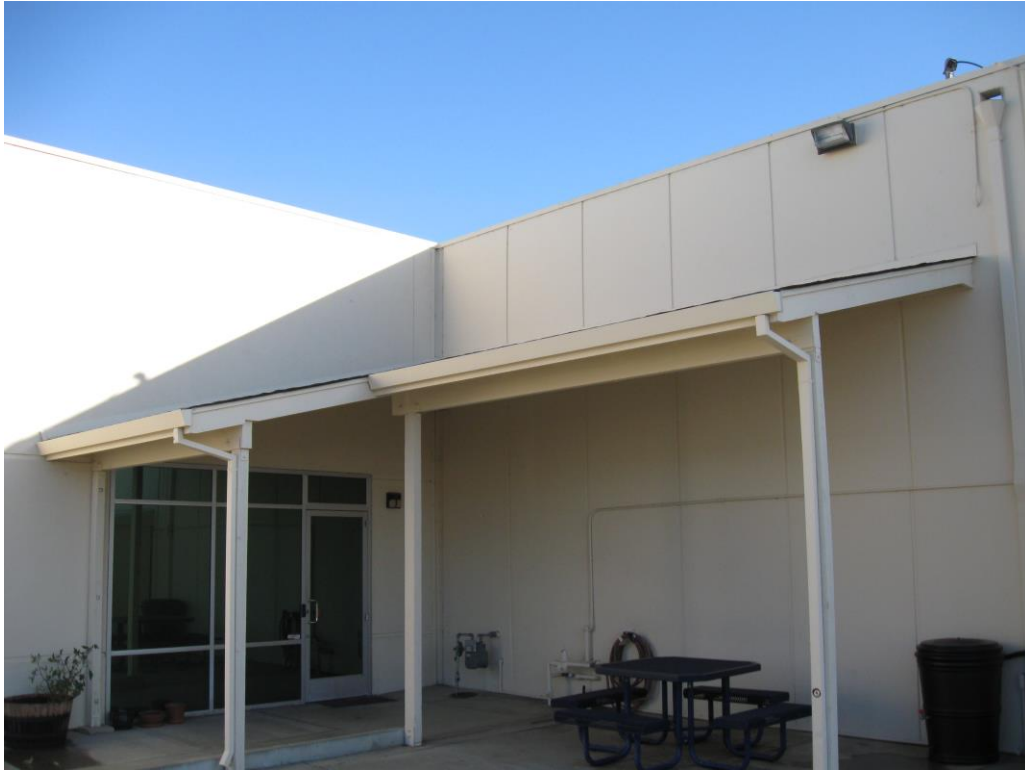
Photo 3: Wood-Framed Canopy Attached to Both Buildings Across Seismic Joint
