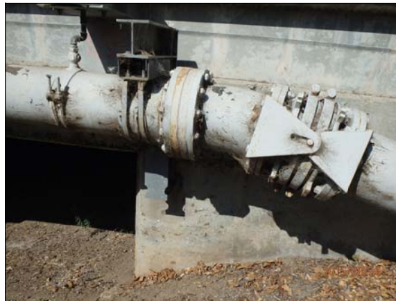
12-INCH TEMPFLEX EXPANSION JOINT (TYP BOTH SIDES) ISLAND PARKWAY BRIDGE
