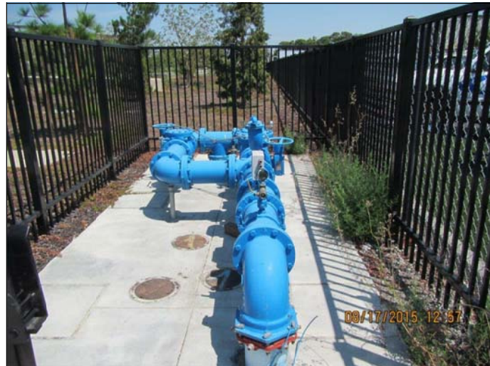
8-INCH CALWATER INTERTIE INDUSTRIAL RD (PAMF)
