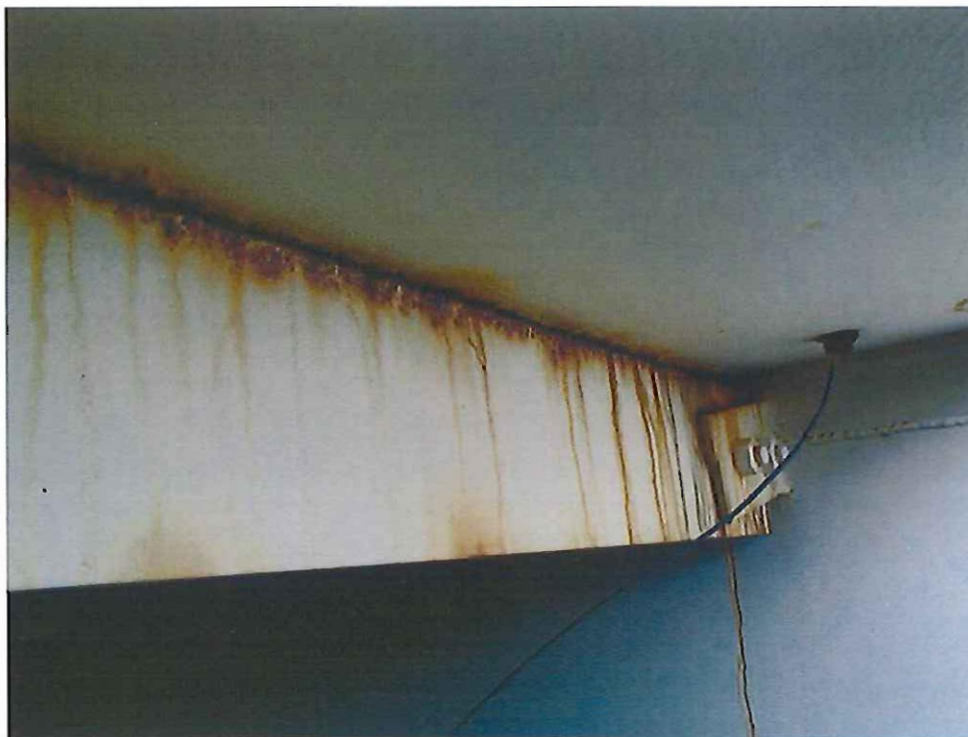
Photo 3: Minor Corrosion at Roof Rafter
