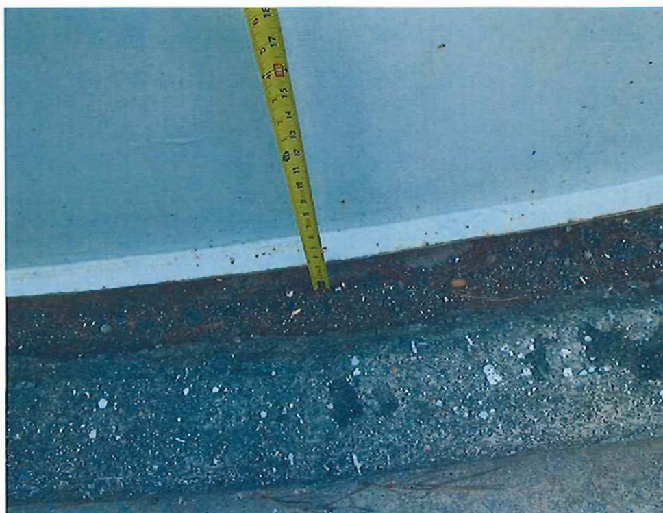
Photo 4: Localized Gaps Below Tank Bottom
