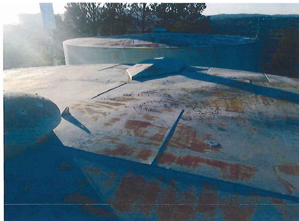
Photo 2: Minor Corrosion of Tank Roof
