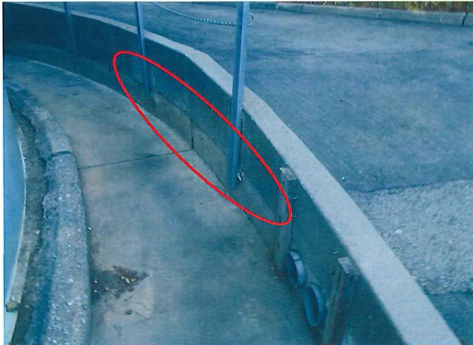
Photo 6: Retaining Wall Addition Adjacent to the Tank
