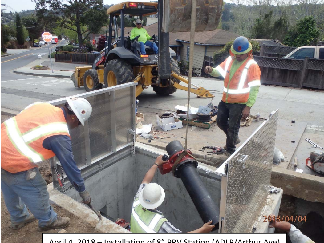
April 4, 2018 – Installation of 8" PRV Station (ADLP/Arthur Ave)
