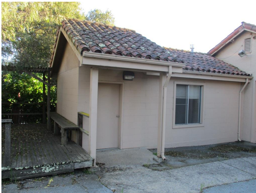
Photo 2: Eastern CMU Building Addition
