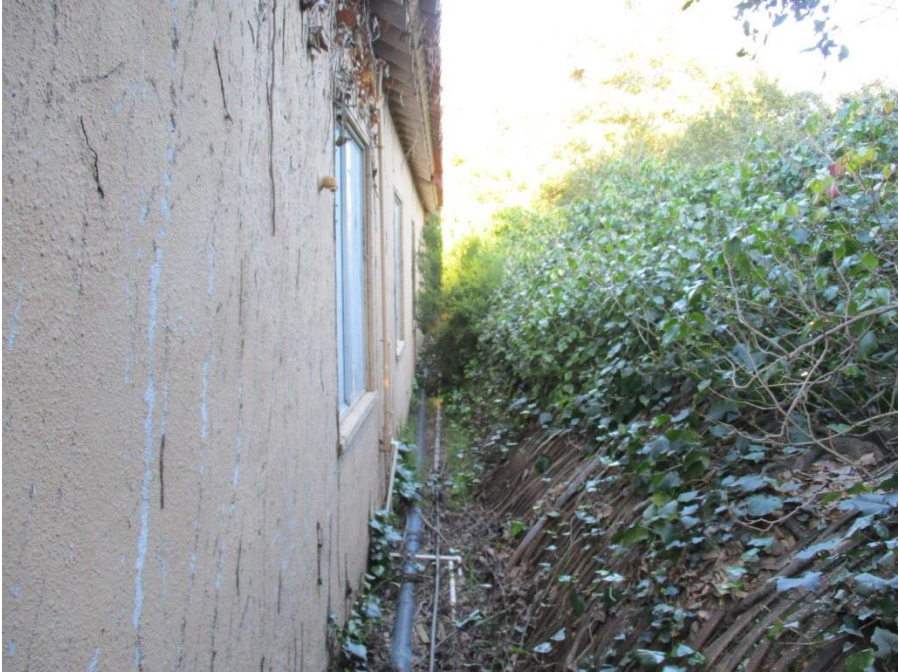
Photo 3: South Building Elevation at Top of Hill
