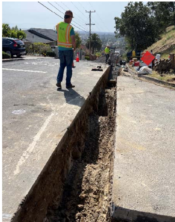
April 27, 2022 – Veins of rock within trench on Vine St.
