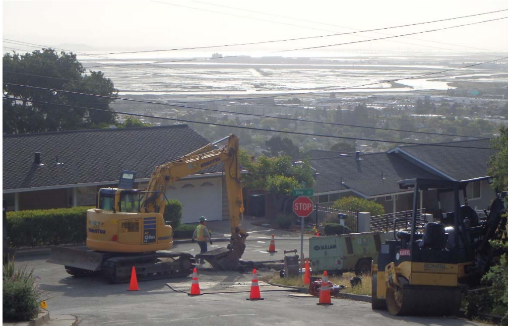
April 27, 2022 – View of Vine St water main installation from Courtland Rd.
