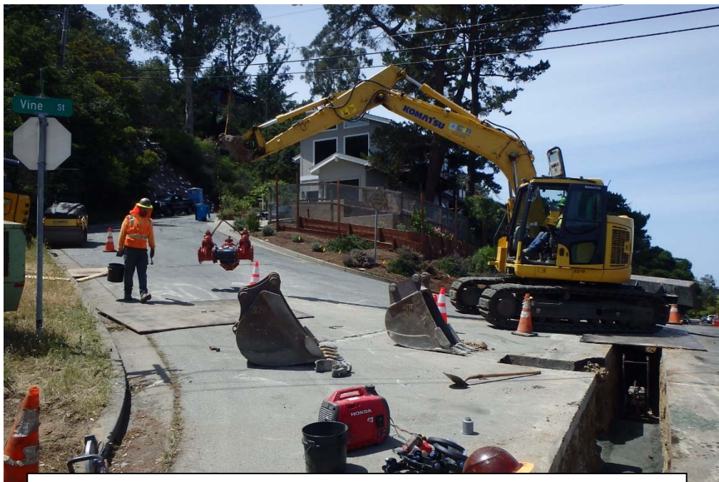
April 27, 2022 – Vine St at Courtland Rd – Installation of 3-valve tee.
