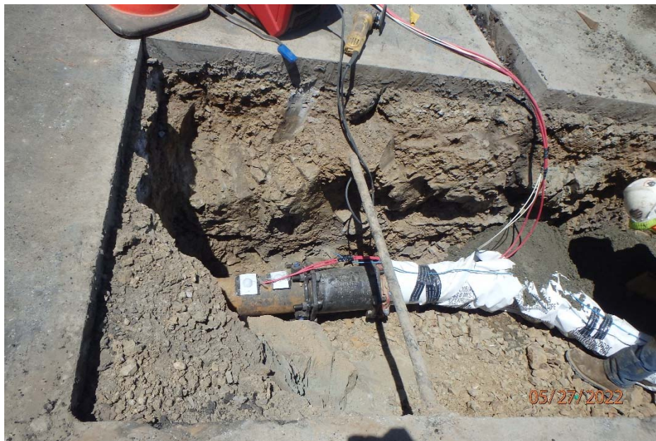
May 27, 2022 – Courtland Road tie-in.
