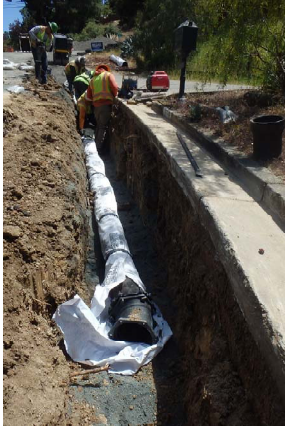
May 10, 2022 – 8” DIP installation along Vine Street.
