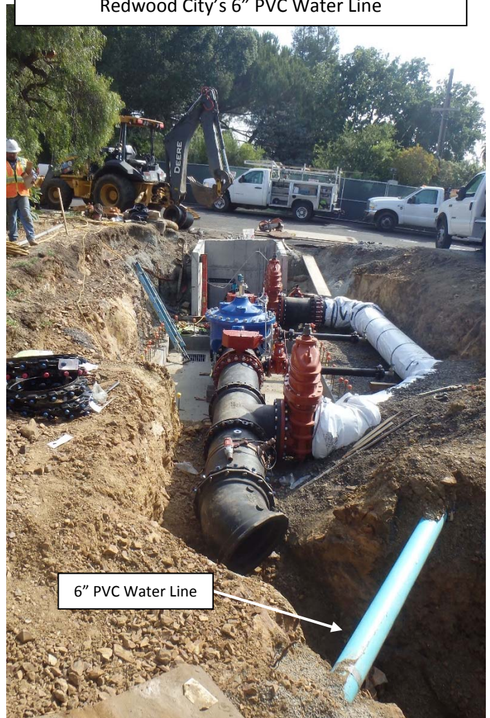
May 29, 2019 – Vertical Alignment Under City of Redwood City's 6" PVC Water Line
