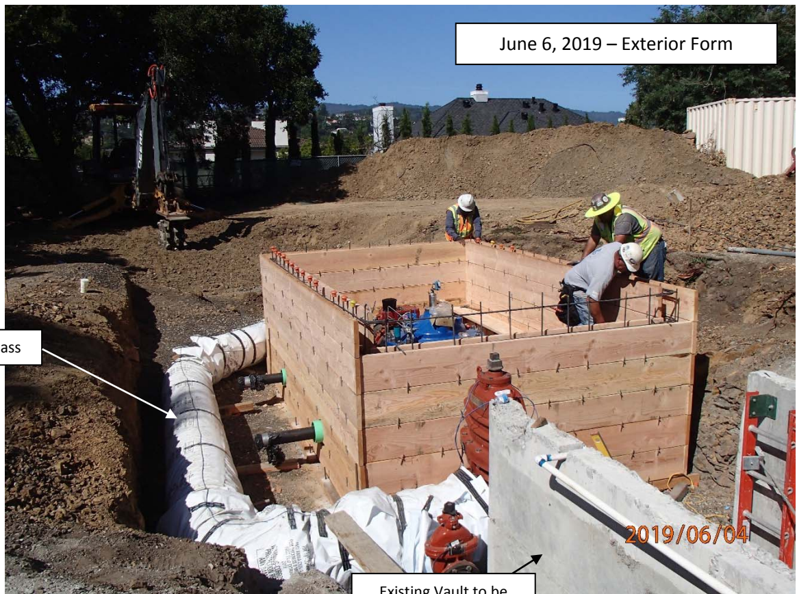
June 3, 2019 – Forming New Vault
