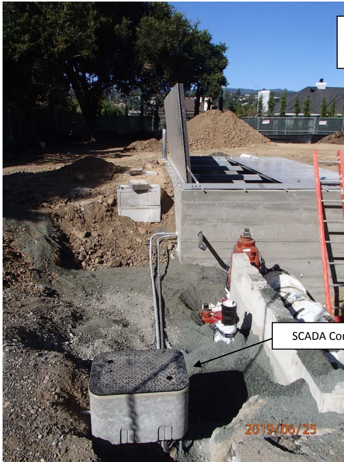
June 25, 2019 – Vault Cover Installation and Electrical Connection
