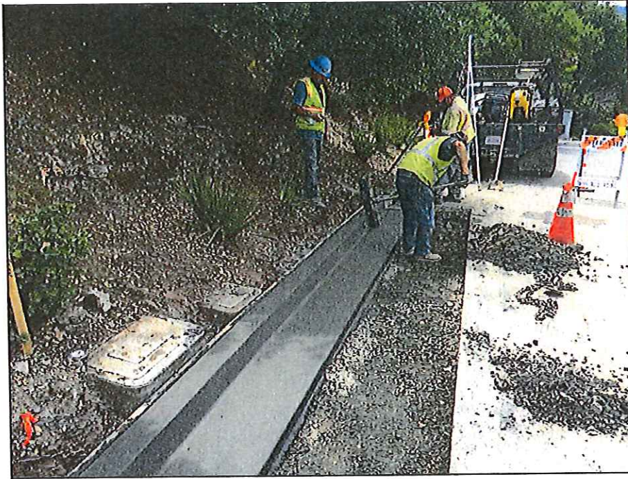
July 2, 2015 - Driveway Curb and Gutter
