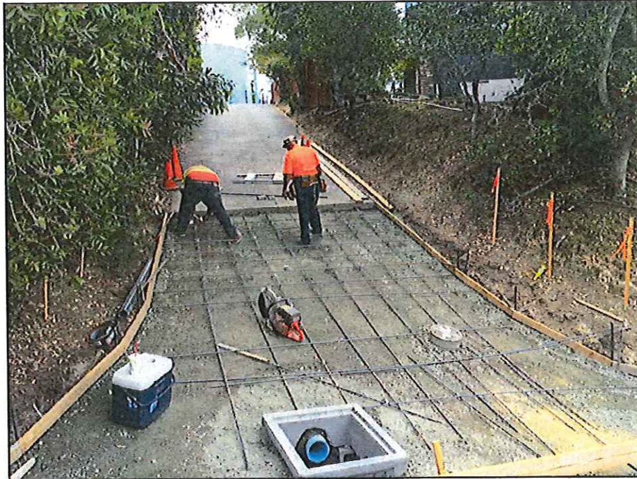
July 1, 2015 - Re-bars and Drain Box
