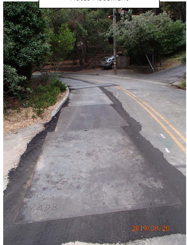
August 20, 2019 – Trench Plates Placement
