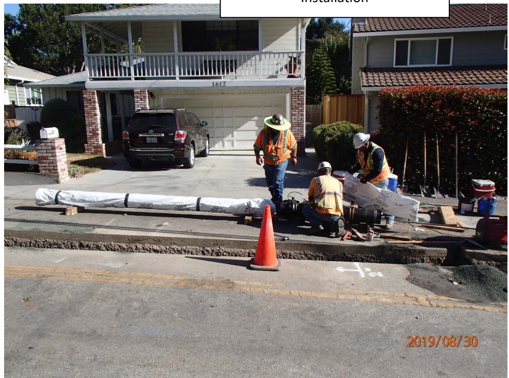
August 30, 2019 – 8" Water Main Installation
