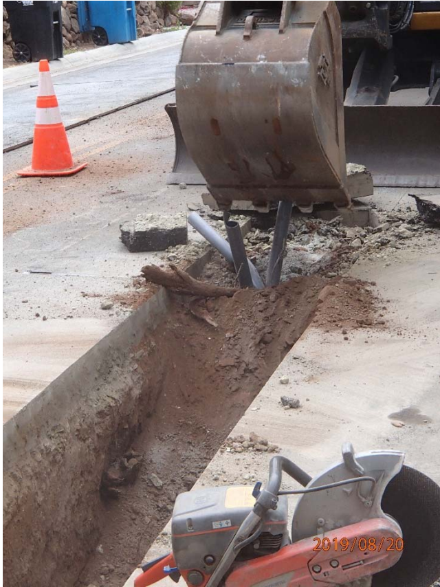
August 20, 2019 – Removal of unmarked 2-2" Empty Conduits
