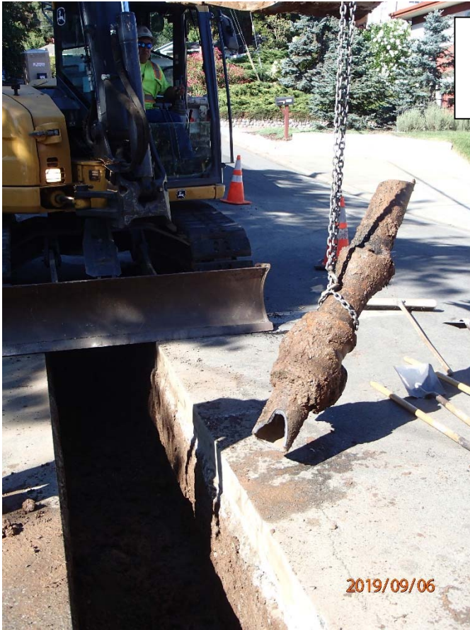
September 06, 2019 – Found the Abandoned 6" Water Main on Valley View Ave
