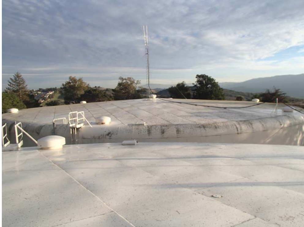
Photo 5: Roof of Hallmark Tanks
