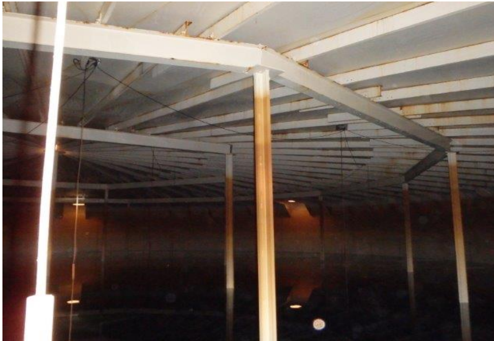
Photo 8: Interior Roof Framing of Hallmark Tanks
