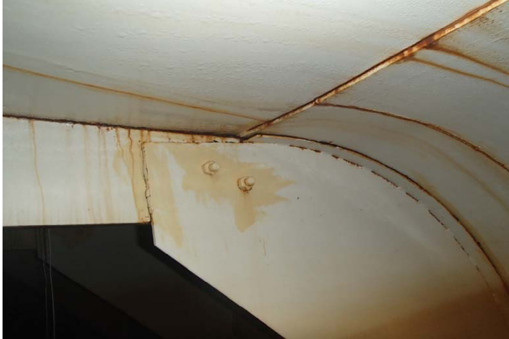
Photo 7: Connection at Roof Knuckle
