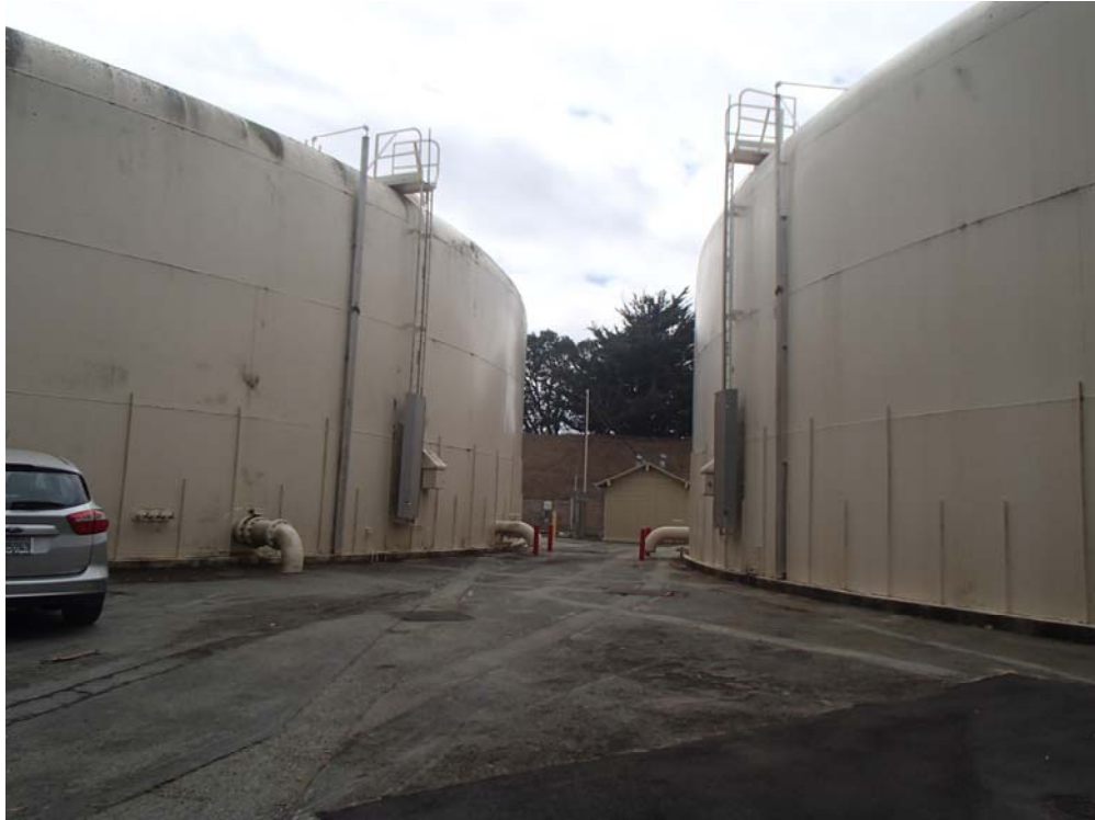
Photo 1: Exterior of Hallmark Tanks
