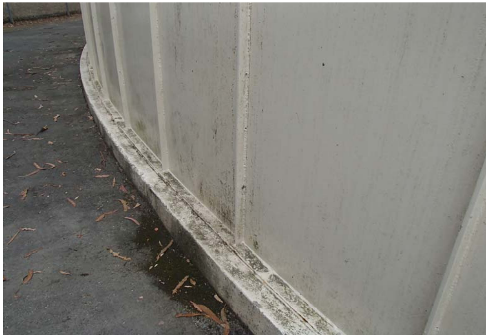
Photo 2: Reinforced Concrete Ringwall Foundation
