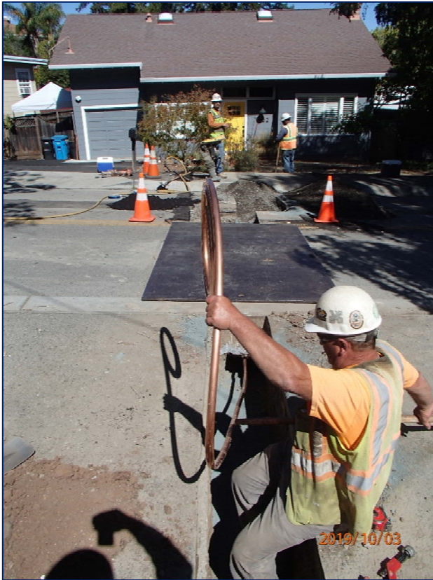
October 3, 2019 – Notre Dame Ave – New water Service Line Connection
