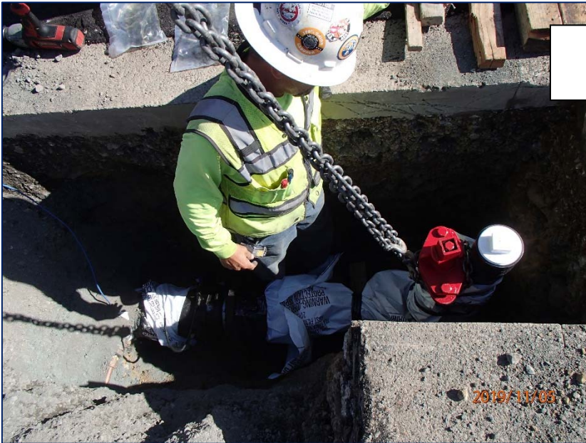
November 5, 2019 – Bryce Ct 4" Blow-Off Installation
