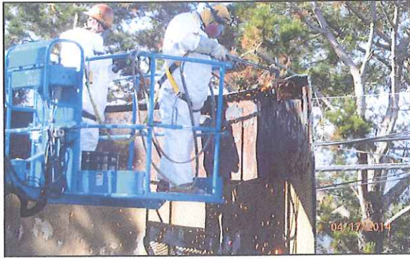
April 17, 2014 - Tank Shell Torch Cutting
