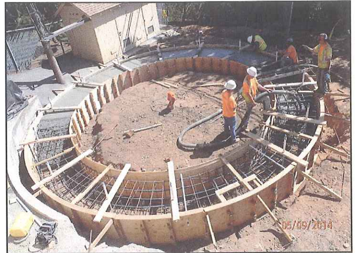
May 9, 2014 - South Tank Concrete Beam Pour
