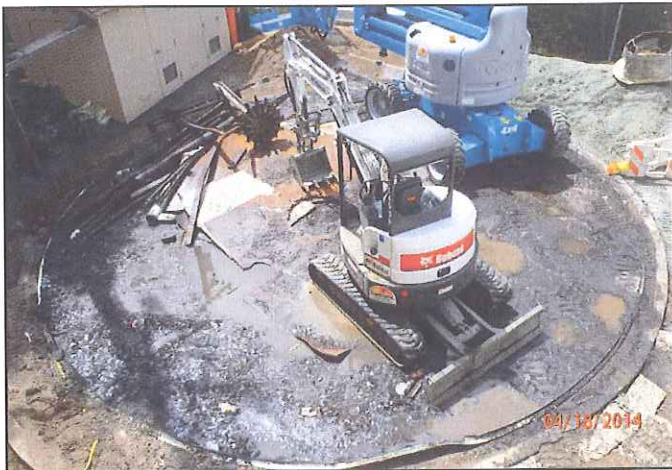
April 18, 2014 - South Tank Shell Demolition Completed
