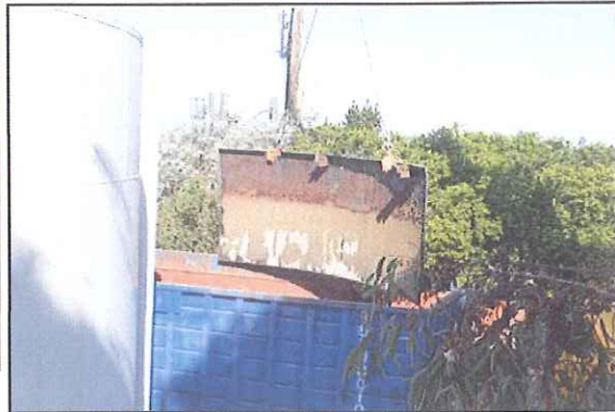
April 17, 2014 - Tank Shell Panel Removal and Disposal
