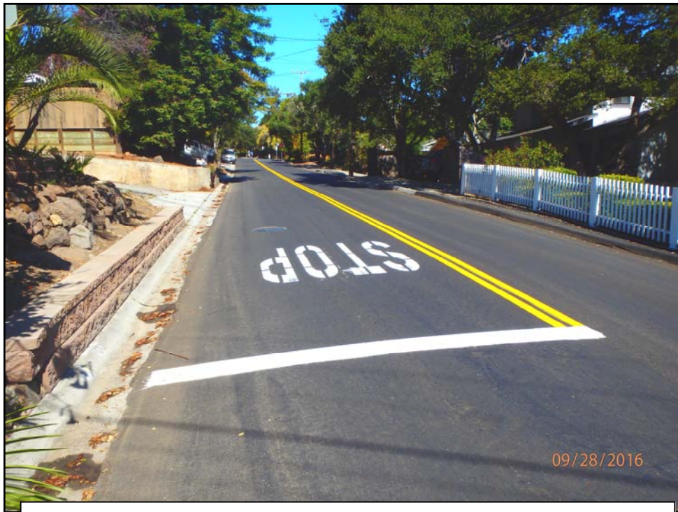
September 17, 2016 - Striping was completed
