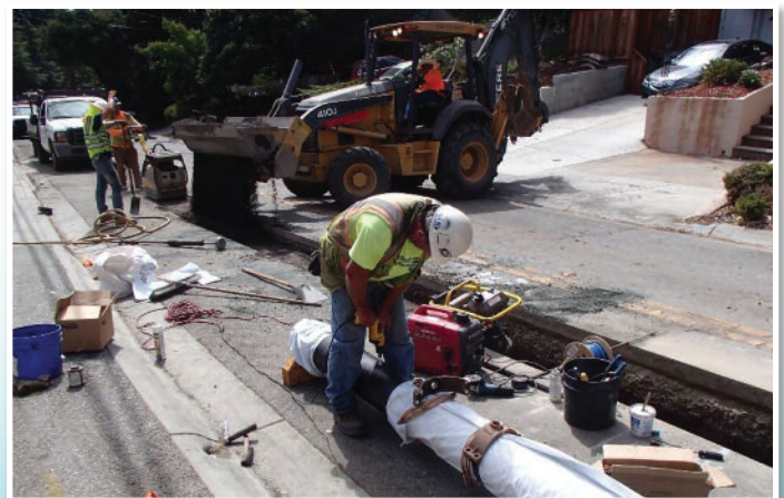
Above: Trenching to install the final 65 feet of water main on Muir Way. Below: Drilling for service connection on Notre Dame Ave.
