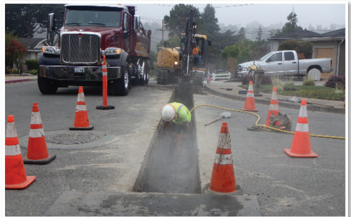
Above: Trenching to install the final 65 feet of water main on Muir Way. Below: Drilling for service connection on Notre Dame Ave.
