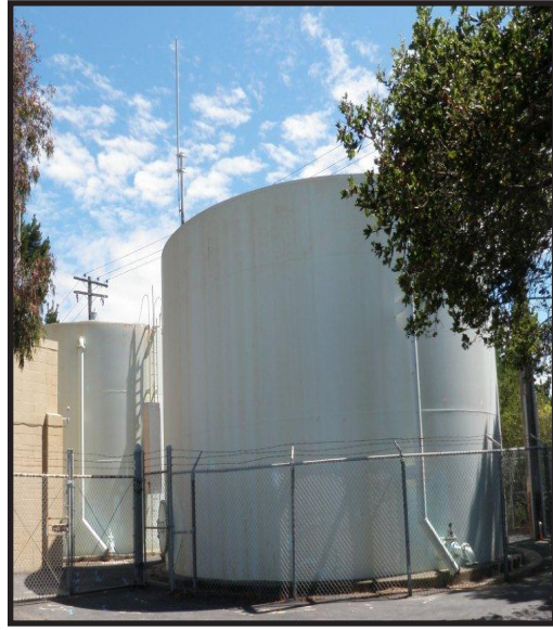
Buckland Tank Site
