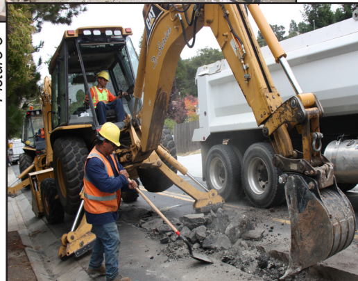
Picture 1- Staff installing new AMI meter Picture 2- Staff repairing a service line leak Picture 3- Staff digging with a backhoe
