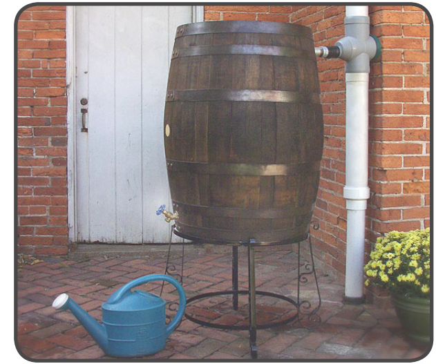
Sample of a rainwater catchment barrel
