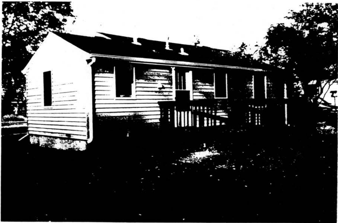
Side and Rear View
