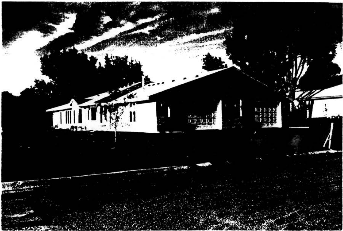
Northeast view of the accessible twin home built at 51st and Winnetka Avenue North.
