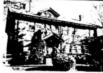
2103 Second Avenue South (housing for the homeless) Alliance Housing Whittier neighborhood, Minneapolis
