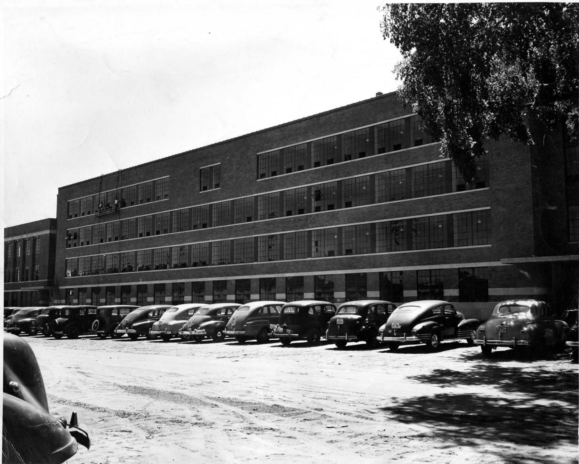
AERONAUTIC ENGINEERING BUILDING UNIV. OF MINN.
