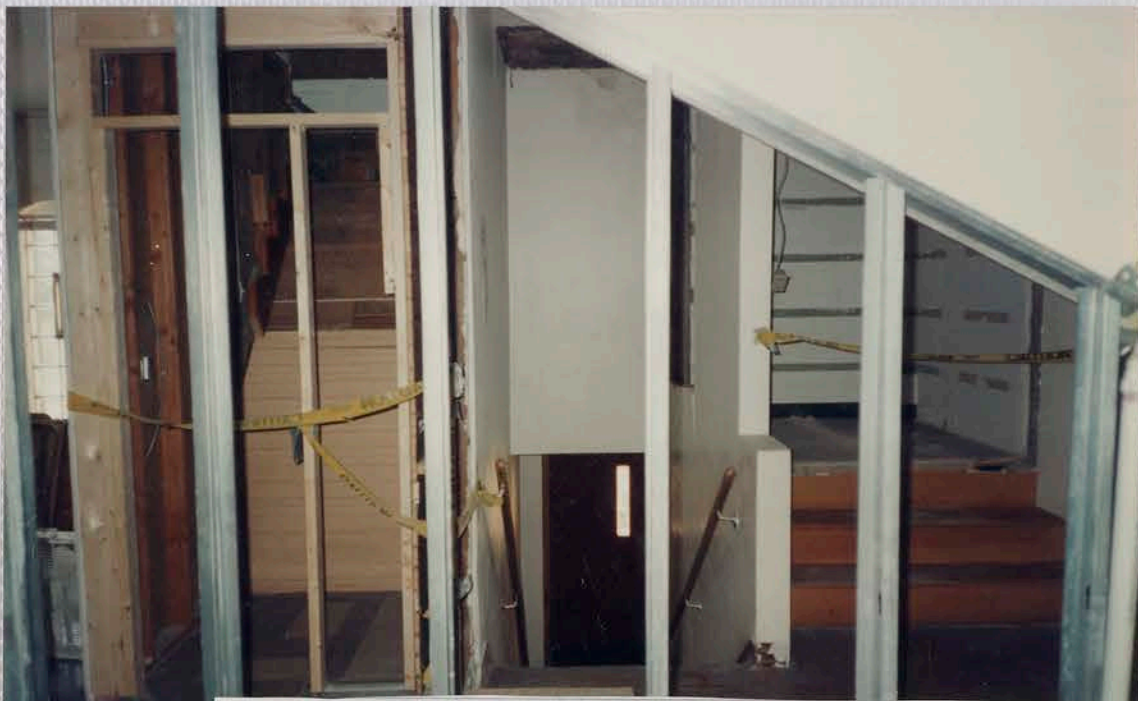
12 During Renovation: Framing new closet and stairway to upstairs
