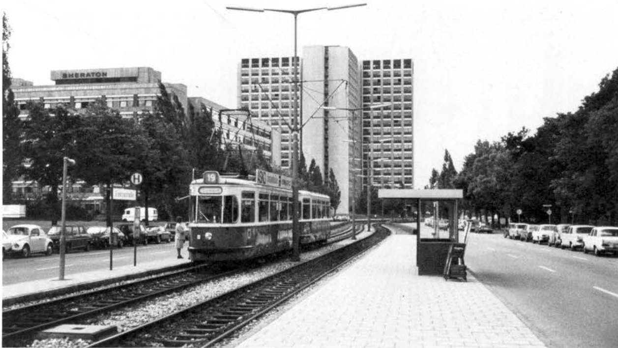
Figure 3. A simple station on a light rail line in the center of a boulevard. Special paving material is used to indicate the station area. The support system for the overhead wires is combined with the street light standards.
