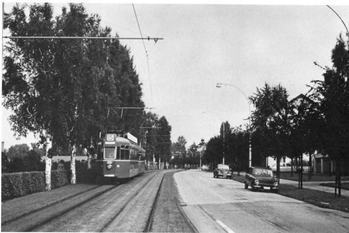
Figure 1. A light rail line on separate right-of-way at the side of a residential street. The right-of-way area is landscaped; the surface is planted with grass.
