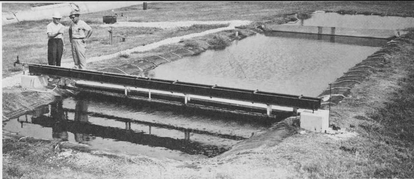
This small, divided pond served as the pilot unit for research on the biological treatment of refinery effluent water at Baytown. Watching are Research Technician Carl Tyler and Research Specialist Sid Brady.
