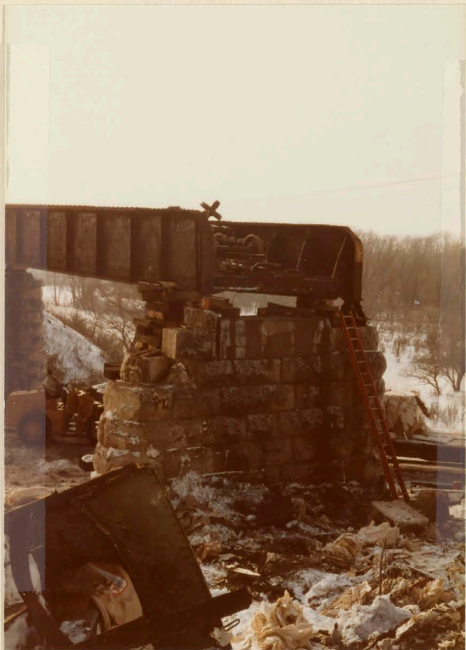
North pier and temporary cribbing
