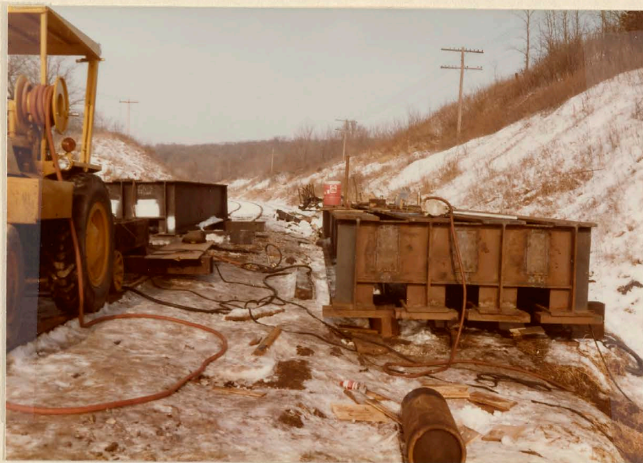
Replacement span for north approach being welded together on site
