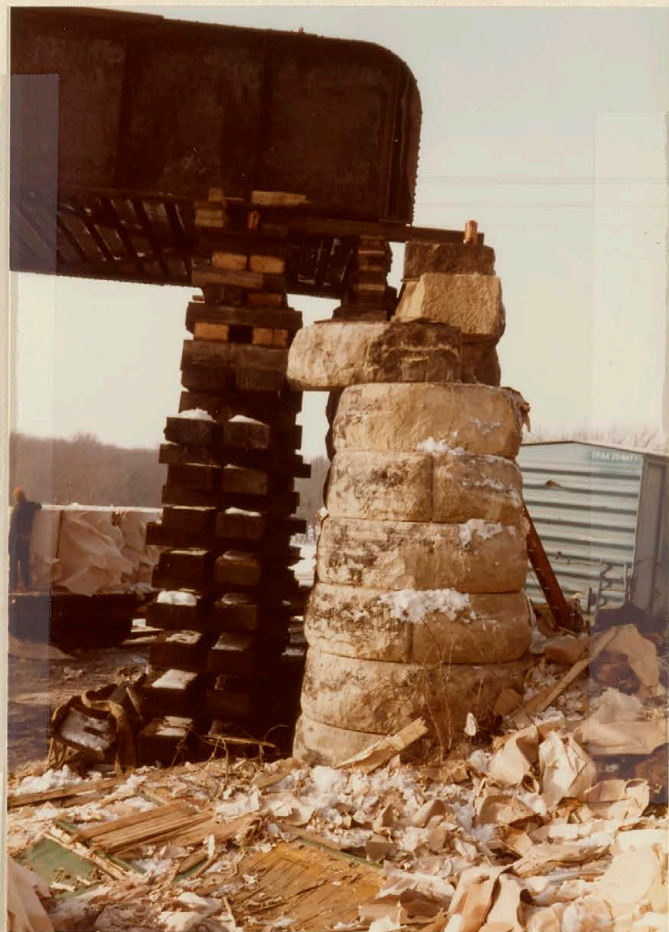
North pier and temporary cribbing
