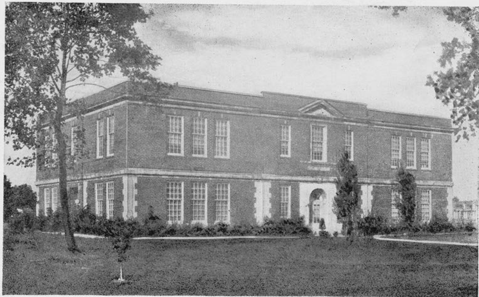
THE HOME ECONOMICS BUILDING, WILBERFORCE UNIVERSITY, WILBERFORCE, OHIO
