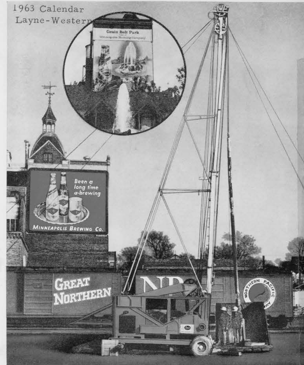
DRILLING "DIAMOND WELL" FOR GRAIN BELT
