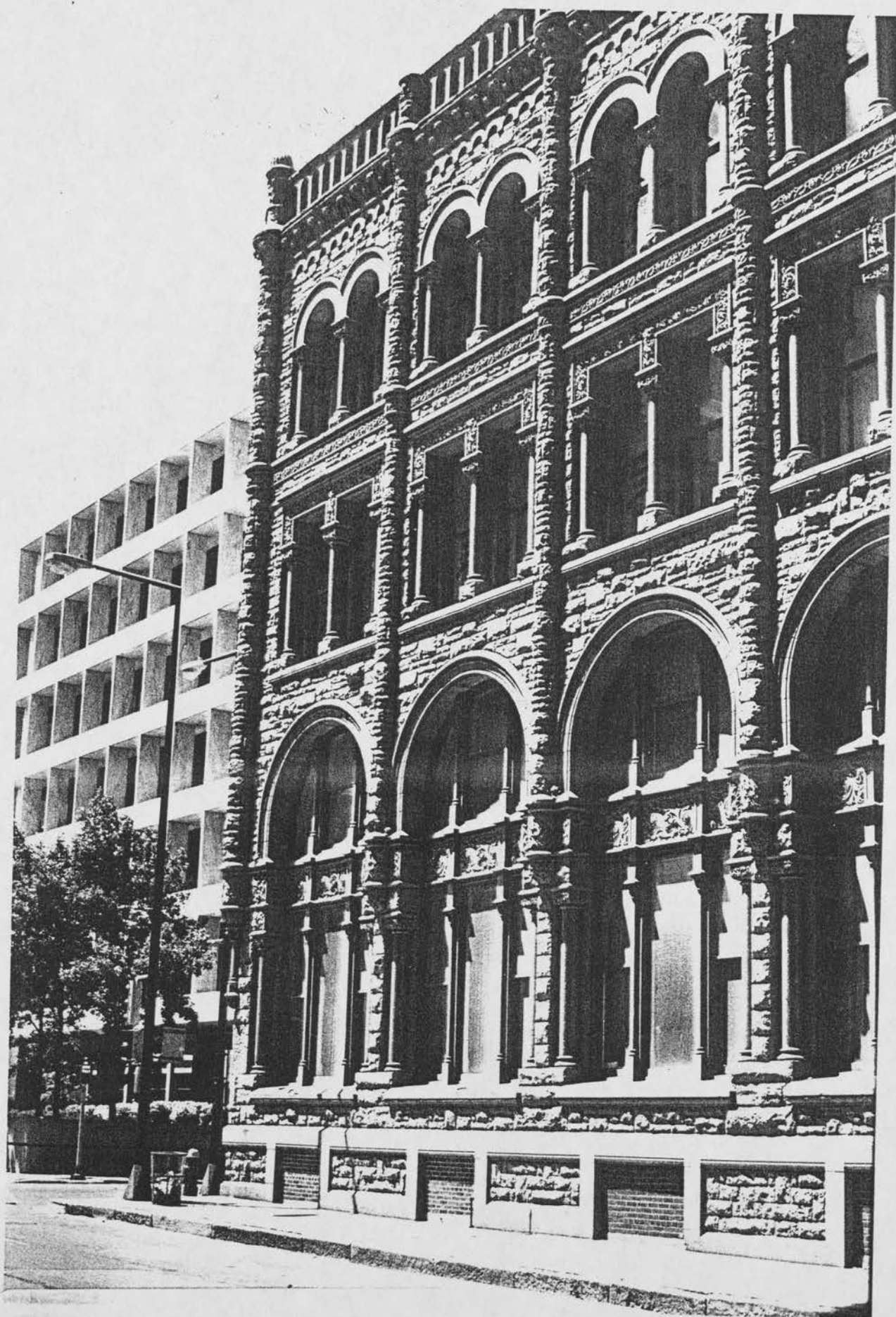
MCCOLL BUILDING FACADE (BLOCK 40)
