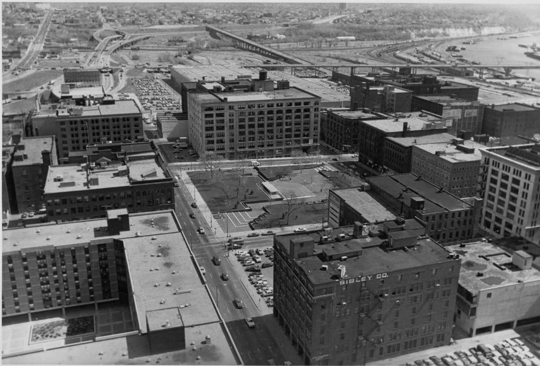
MEARS PARK (pre-construction of — (Block 40, and restoration of Finch, — Parkside, and Globe-Rosenthal Bldgs.
