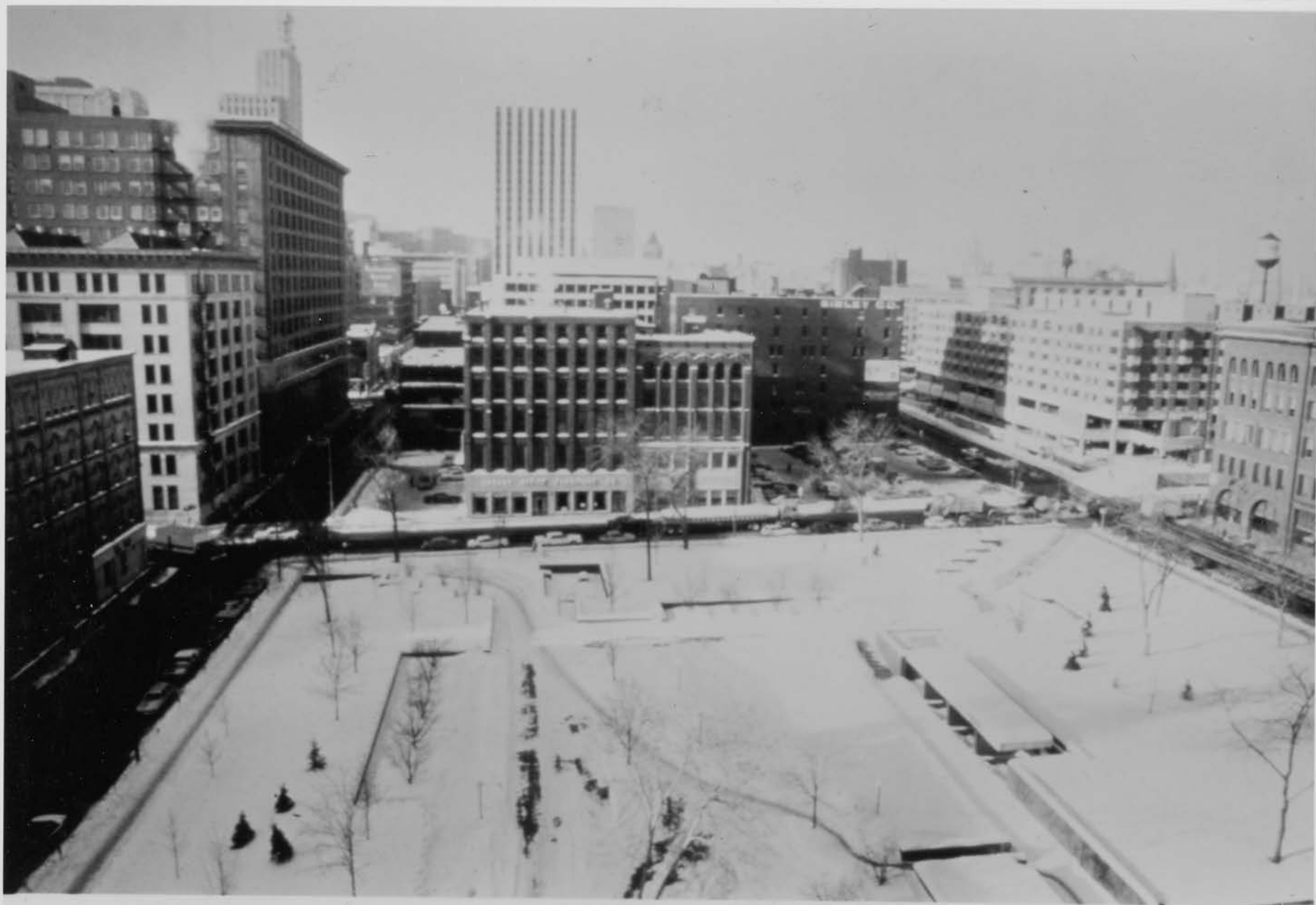
MEARS PARK (pre-construction of — Galtier Plaza—Block 40)
