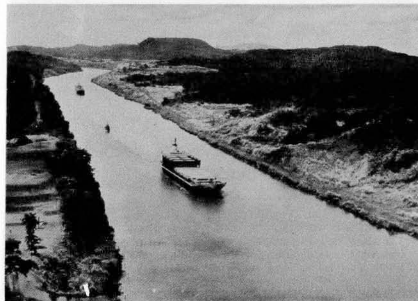
Above: Container ship "Elba Maru" moves through a narrow section of Gaillard Cut, which has been widened over the years from 300 to 500 feet to increase safety and permit greater two-way traffic. Below: Traffic moves easily through the widened channel.
