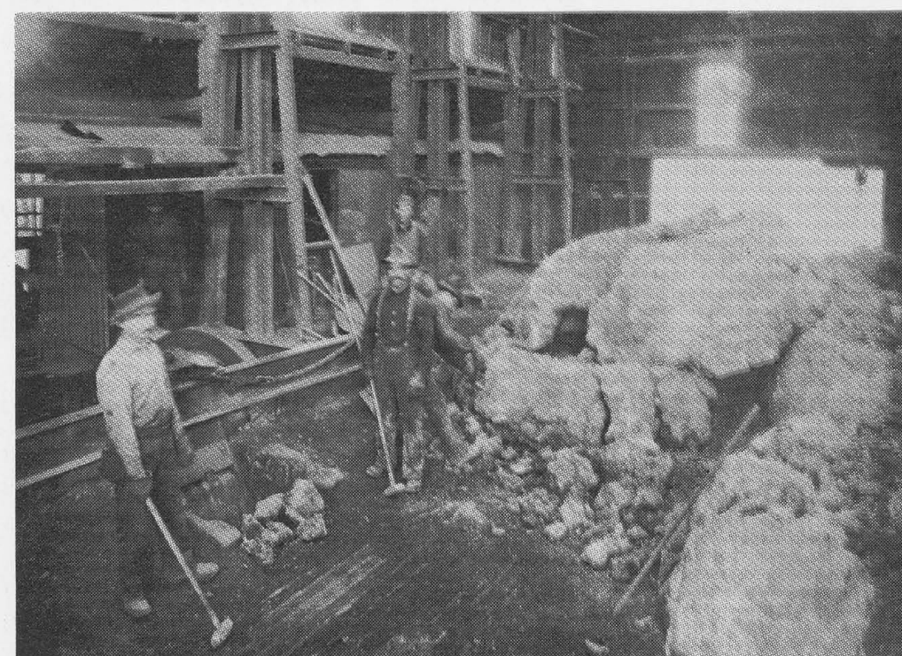
This is a vivid representation of the time consuming, back-breaking and expensive task of breaking up the product of the batch roasting processes in use before continuous sintering.
