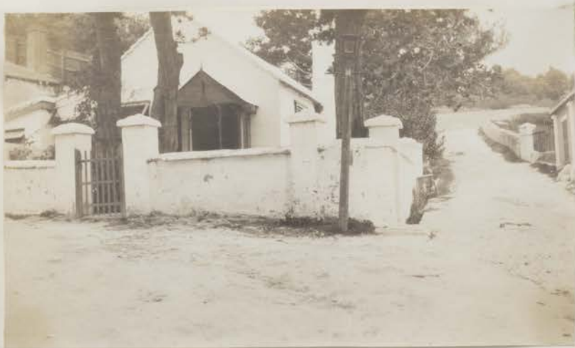
An old house at St. George
