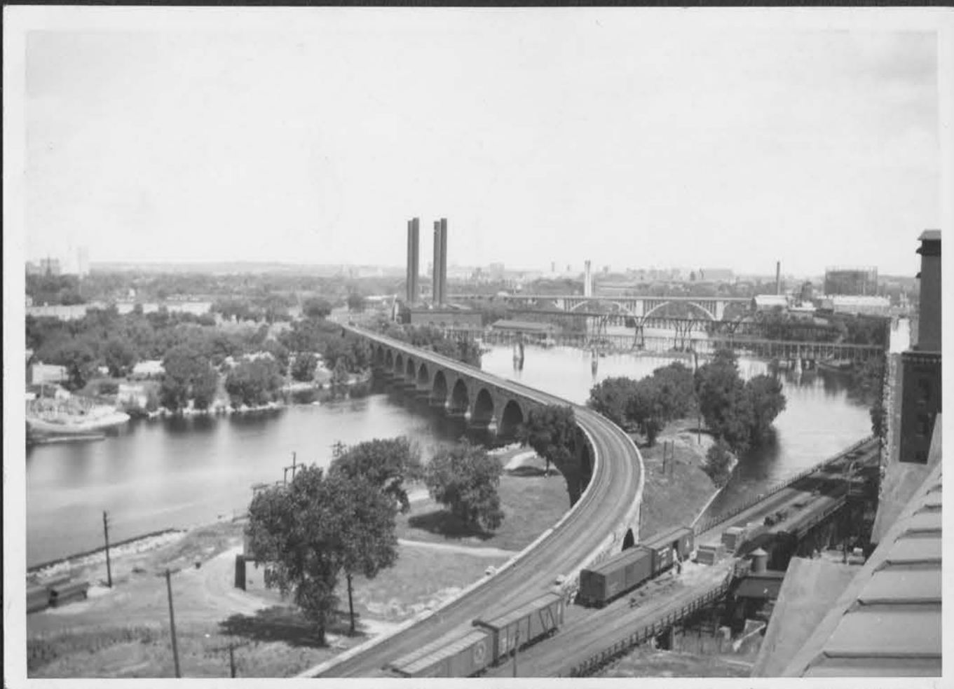
BRIDGES - MISSISSIPPI RIVER MINNEAPOLIS - MINNESOTA
