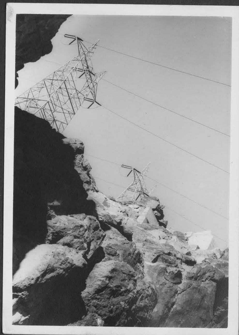
TRANSMISSION TOWERS NEVADA
