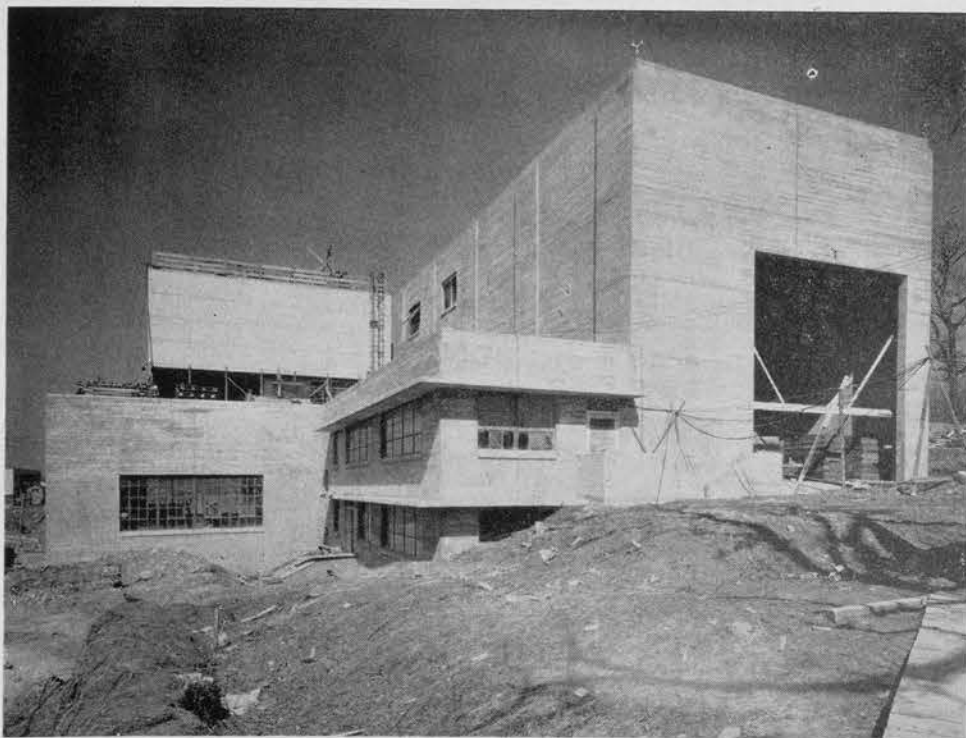
Top of page, an early wind tunnel at an Army air field, designed by the Constructing Quartermaster Corps. Lower picture shows the cold chamber for a wind tunnel; here are included a large testing area, office and control room space, and a refrigerating unit. This unit was designed by J. Gordon Turnbull, Inc., and Sverdrup and Parcel, consulting engineers. (Official U. S. Army Air Corps Photos.)
