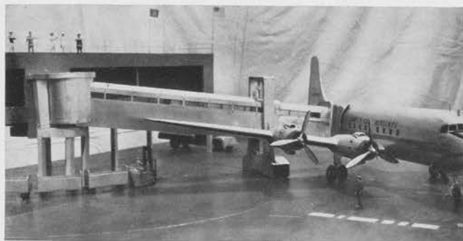
Mobile, covered gangplanks, as developed by the Airways Engineering Corp., provide protected passenger loading from finger to plane (above). Fewer apron positions are required, and more passenger miles may be flown, since loading time is reduced.
