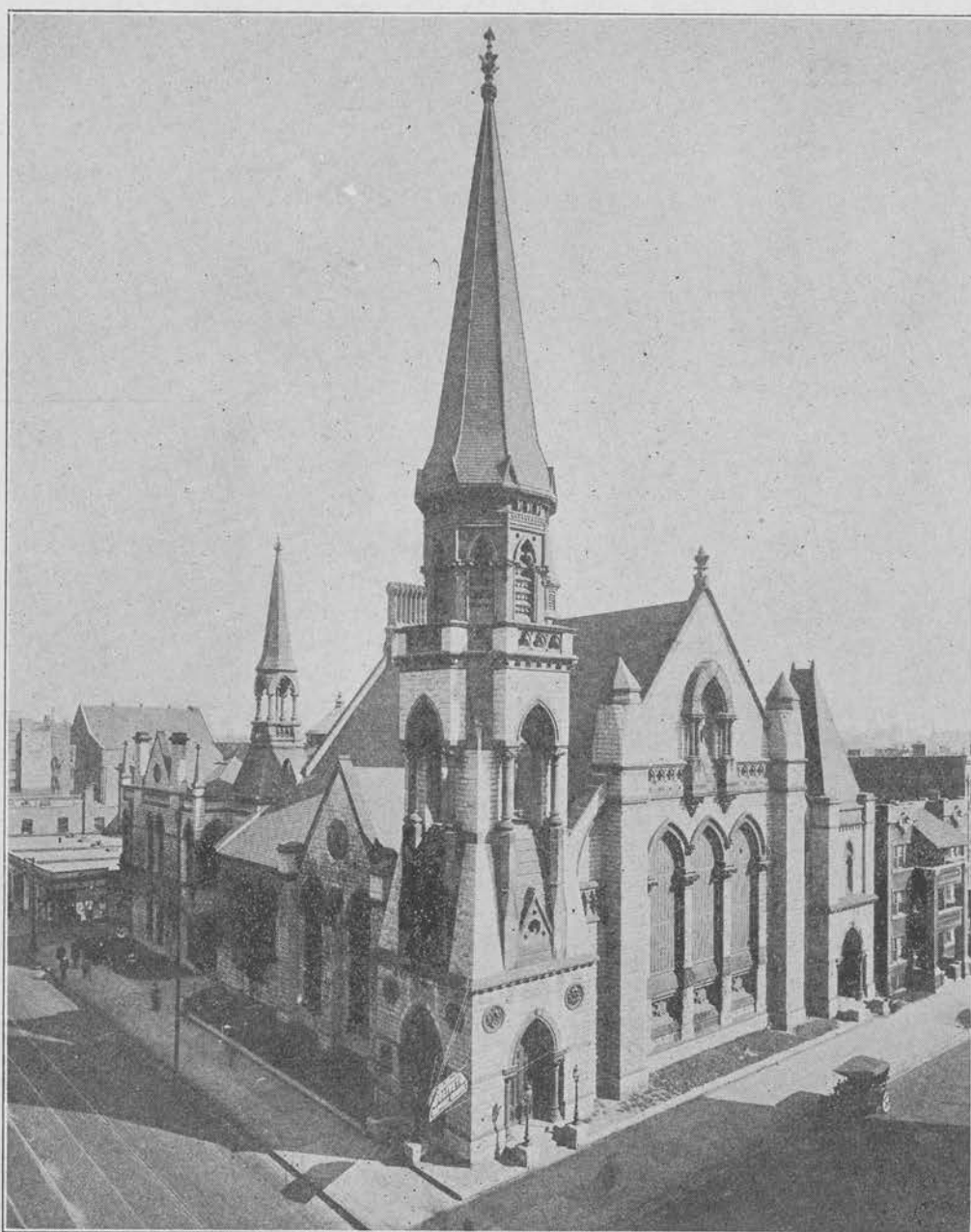
OLIVET CHURCH, CHICAGO, FORMERLY HOME OF THE FIRST CHURCH.
