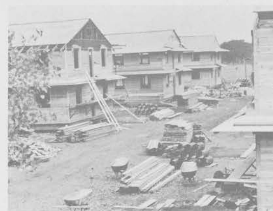
Reception center barracks under construction in 1940
