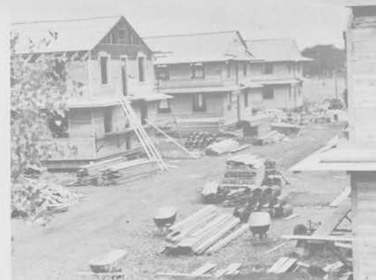
Reception center barracks under construction in 1940
