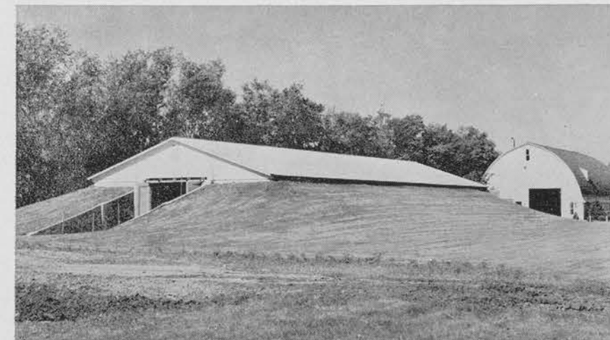
Tree storage and workshop, Oakes Nursery.
