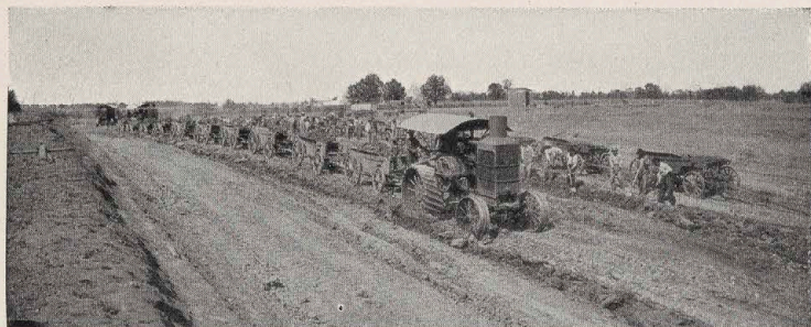
Hart-Pan tractors used in early construction work on Great Northern Ry.
