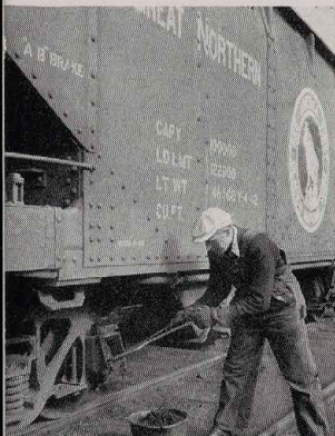
This "ground crewman" is oiling the bearing on which a car wheel rolls. Oil-soaked waste lubricates the bearing.
