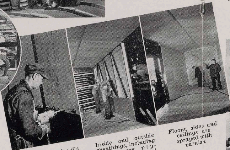
Steel bolts and nails are used to hold the plywood sheathing in place
