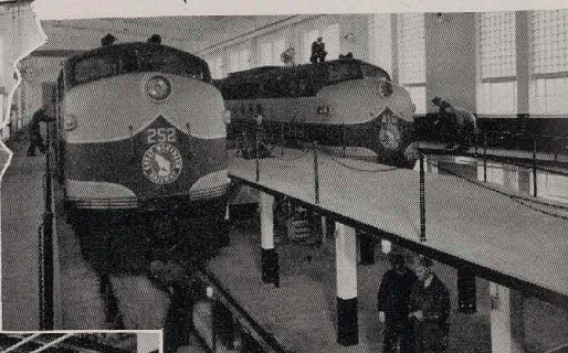
Elevated concrete platforms provide working areas at same level as locomotive floors
