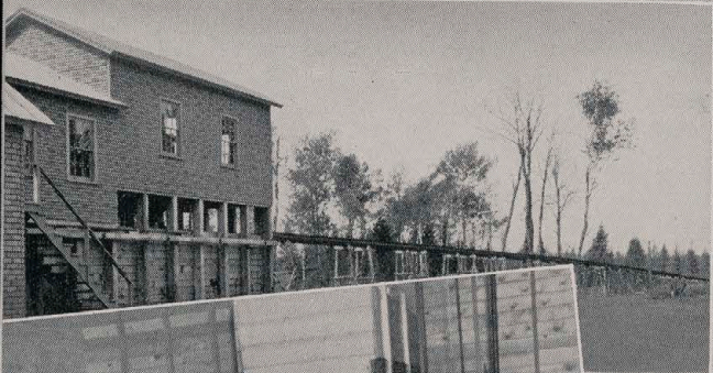
Wet peat is pumped through 800-feet of eight inch pipe into a screening room where all debris is removed.
