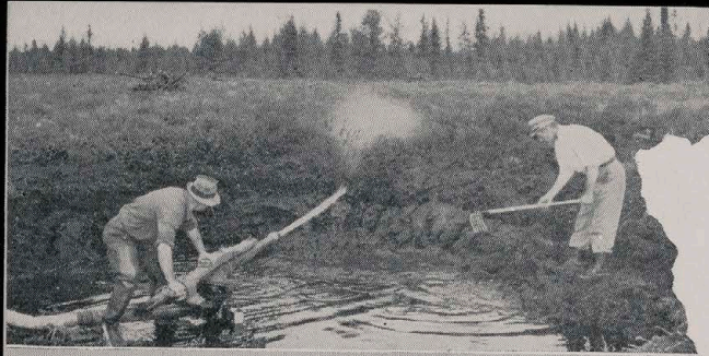
A hydraulic pressure hose forces the wet peat from the bog and down a sluice.
