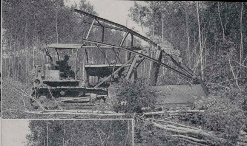
Land clearing is rapidly done by mounting a V-shaped blade on the front of a giant caterpillar.
