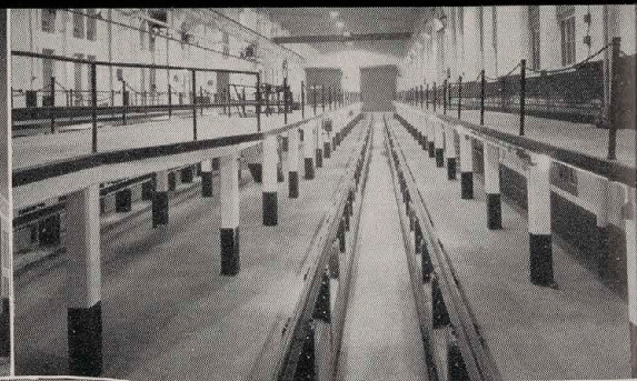
Steel column supports for the 205-foot service track pit rails facilitates the work of men in the pits and provides improved lighting
