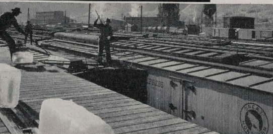
Refrigerator cars are pre-cooled to insure apples arriving at markets in prime condition.
