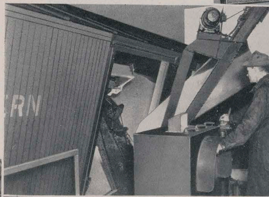
As the metallic arm grips the wooden grain door and pushes it back into the car, the grain cascades into the pit below.
