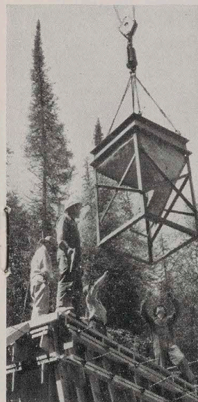
Left: Two yard buckets carry concrete from across the Flathead River for construction of bridge piers. Eight yard buckets will be used for pouring concrete for Hungry Horse Dam.
