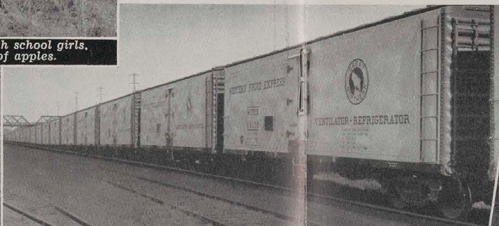
Completely modern refrigerator cars, with steel exteriors, transport Wenatchee apples to markets across the nation.
