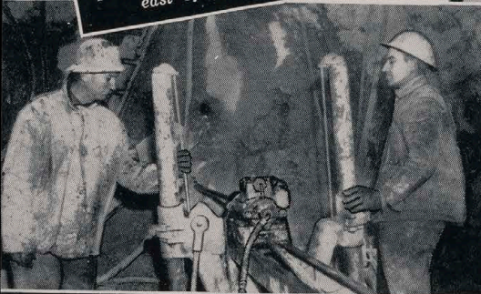
Wagon drill crews drill powder holes into rock, largest winter-time job at Hungry Horse Dam.
