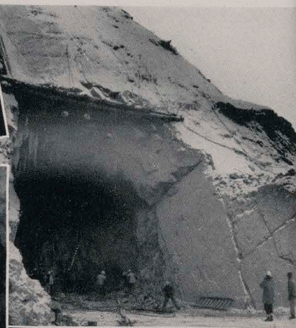
Outlet of 1,100 foot long, 36-foot in diameter tunnel through which south fork of Flathead River will flow while dam is being built.
