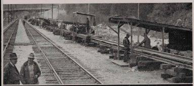
The Oxweld "assembly line" at Scenic Washington, where the heavy 39-foot rails are welded into continuous 1326-foot lengths.
