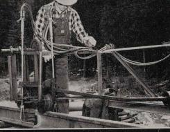
Mill scale is removed by intense heat, then special corrosion-resistant primer is applied.
