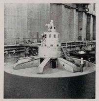
First generating unit completed in East Powerhouse at Grand Coulee Dam.
