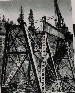
Ninety-six foot girder for center span of new bridge is locked into position with temporary diagonal support in place.
