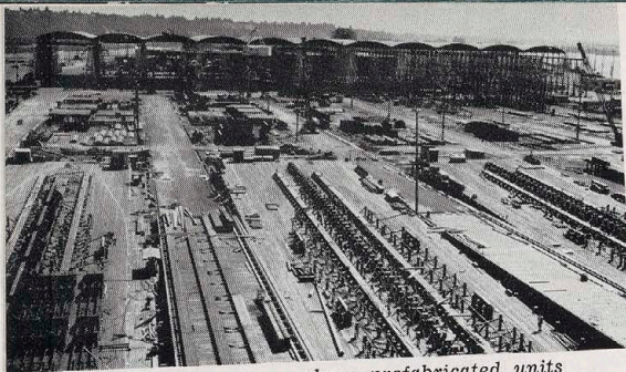
Assembly area from where prefabricated units are trucked on trailers or carried by traveling cranes to the assembly storage areas in front of the ways.
