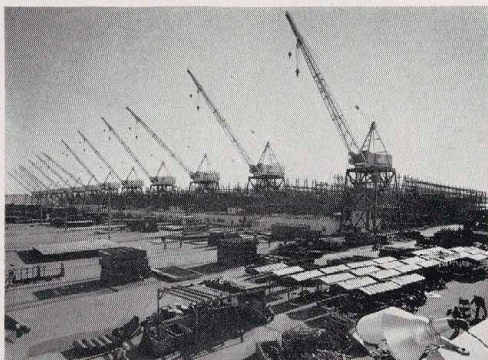
By the time a keel is laid for a vessel most of the assembly units are waiting to be installed and are lifted into place by forty-ton "whirley" cranes and welded immediately.
