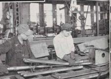
Combination weld backing copper bar frame being inserted into bolster section.
