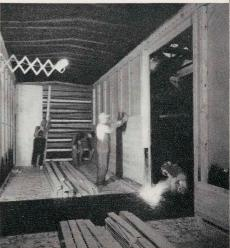
Steel sides, ends and top in place, lumber lining is installed in new cars.
