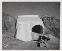
The main canal of the Columbia Basin Project will discharge through this inlet structure into the completed barrel of the Bacon Siphon which disappears into the ground.
