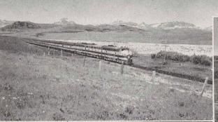
First segment of old line eliminated by Spotted Robe-Triple Divide relocation. New line segment (in background) is built on fill.
