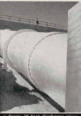
a dozen 12-foot discharge pipes ich carry water 280 feet out of the Columbia River.
