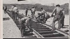
Final spiking job is completed by crew with gasoline-powered spike driver.
