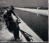
Water flows from the main canal through control gates to lateral canals, thence to fields.
