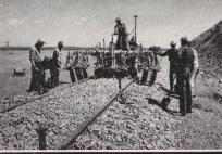
Self-propelled multiple ballast tamper was used for tamping of crushed rock ballast.
