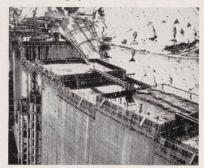
Concrete placement at Hungry Horse Dam in Northwestern Montana has reached 434 feet above bedrock.
