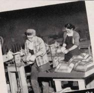
Small machines used to form the "beading" on adjustable galvanized elbows.
