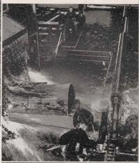
Differing from wood, bark does not dissolve so is removed by hydraulic pressure. Seattle Times photo.
