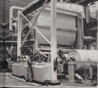
new paper machine makes a ton-and-ajalf jumbo roll which is cut into three curent rolls on rewinder. Times photo.
