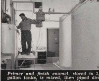
Primer and finish enamel, stored in 3,000-gallon tanks, is mixed, then piped directly to spray equipment.
