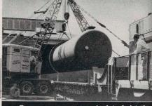
Four cranes were required to hoist the 125,000-pound high pressure autoclave onto GN flatcars.
