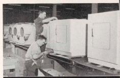
Nearly completed clothes dryers move toward the end of the assembly line.
